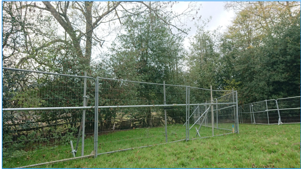
Typical tree protection barrier construction
