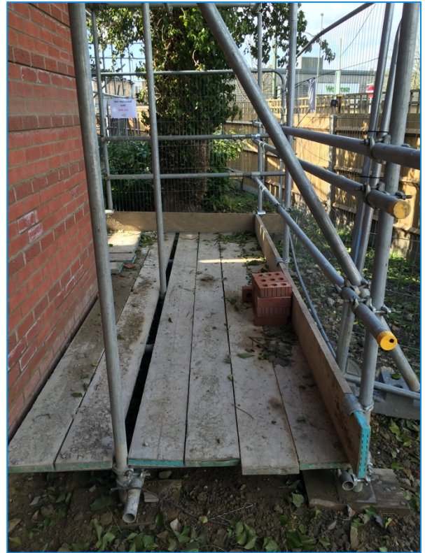
Scaffold ground protection
