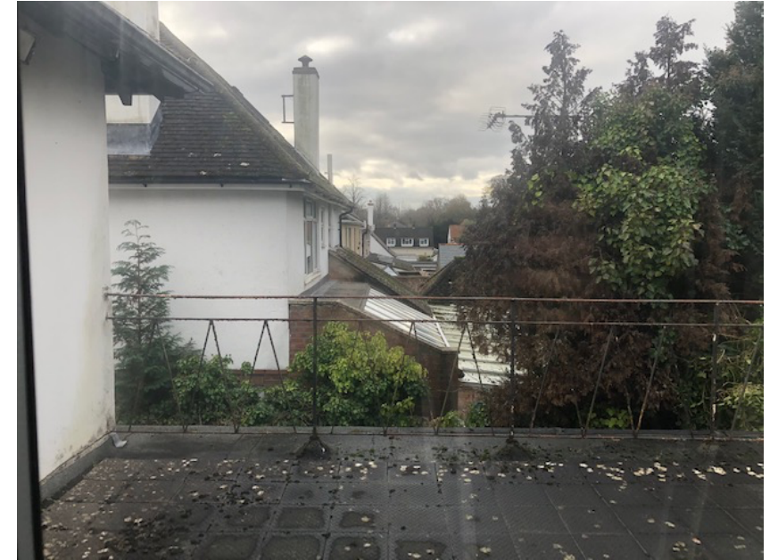
Photo of existing handrail
