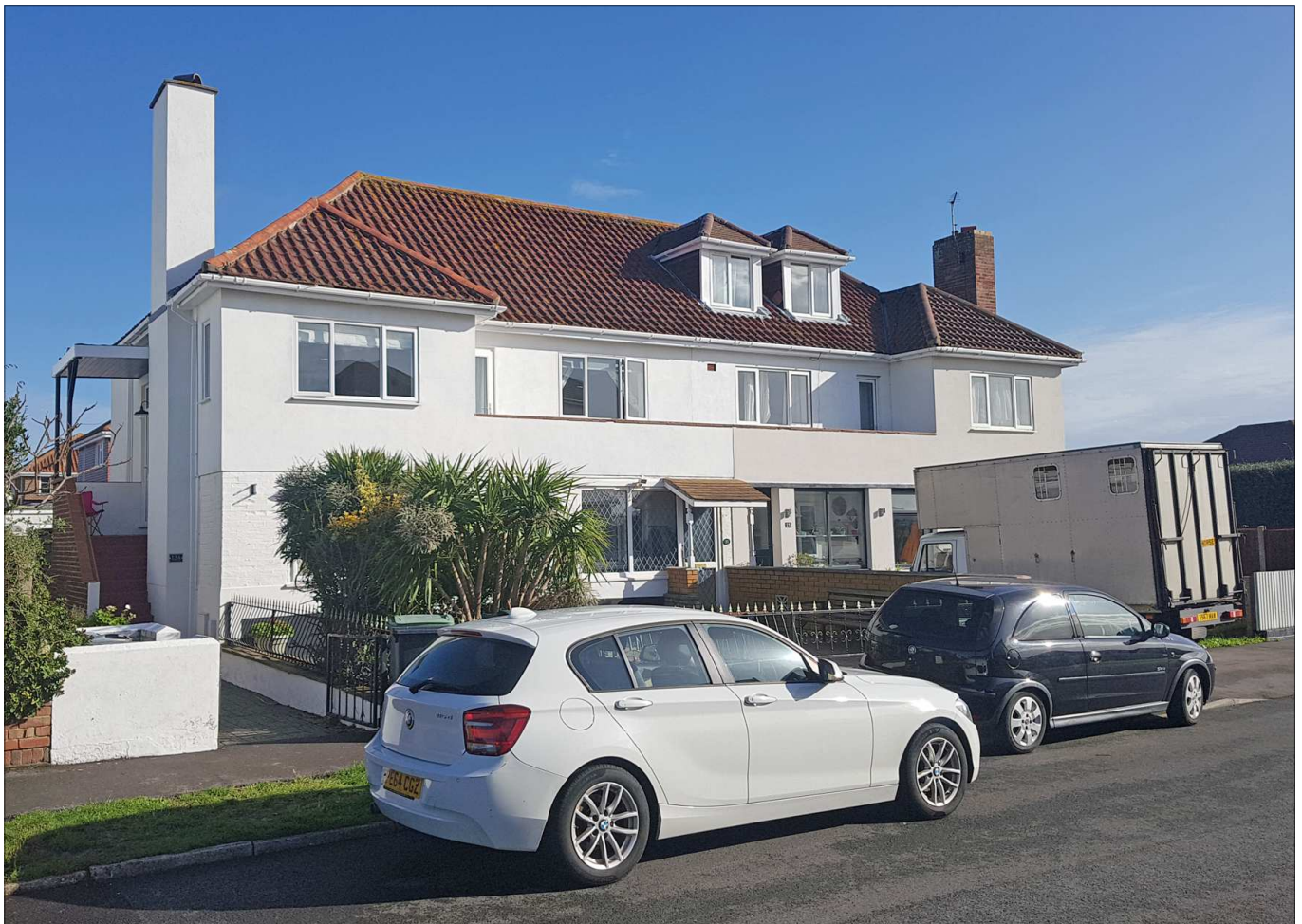
Front of No. 13 & 13A Bembridge Drive (left) and 15 & 15A Bembridge Drive (right)
