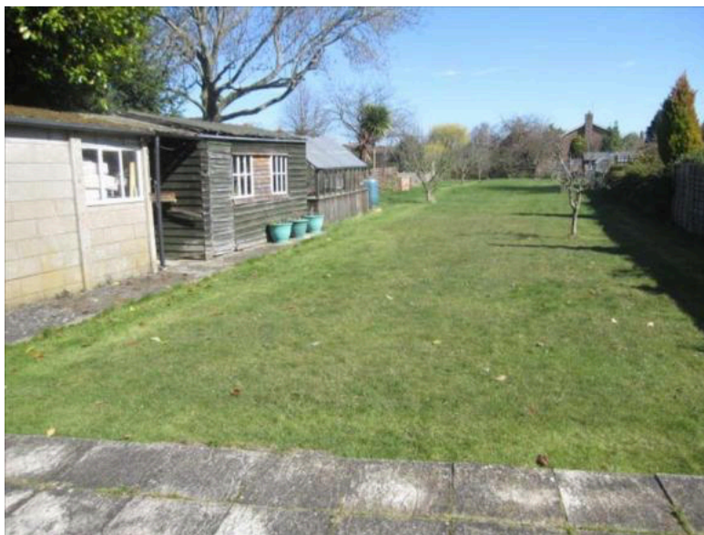
The old sectional concrete (prefabricated) garage and the existing garden shed (south elevation)
