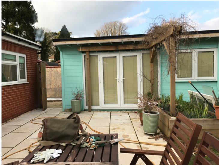
South elevation of the timber garden building
