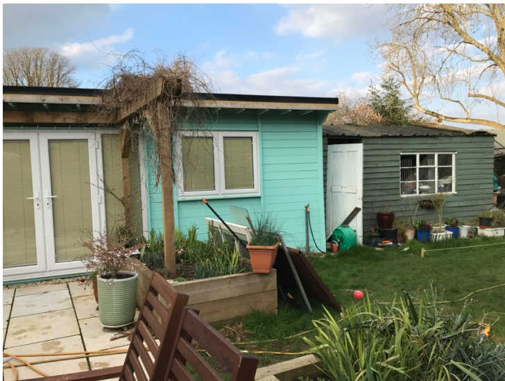
South elevation of the timber garden building and garden shed
