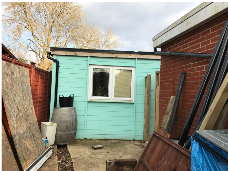
West elevation of the timber garden building
