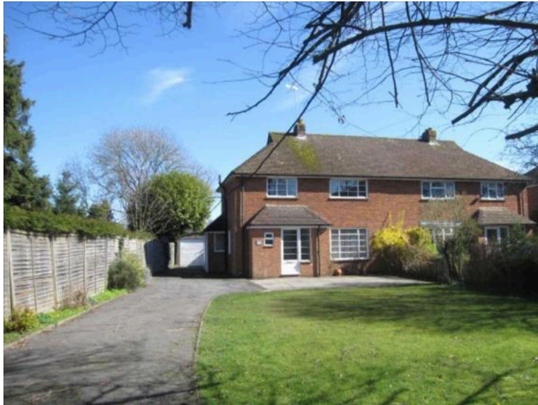
The old sectional concrete garage, which was closer to the boundary with the adjacent property than the replacement timber shed (west elevation)
