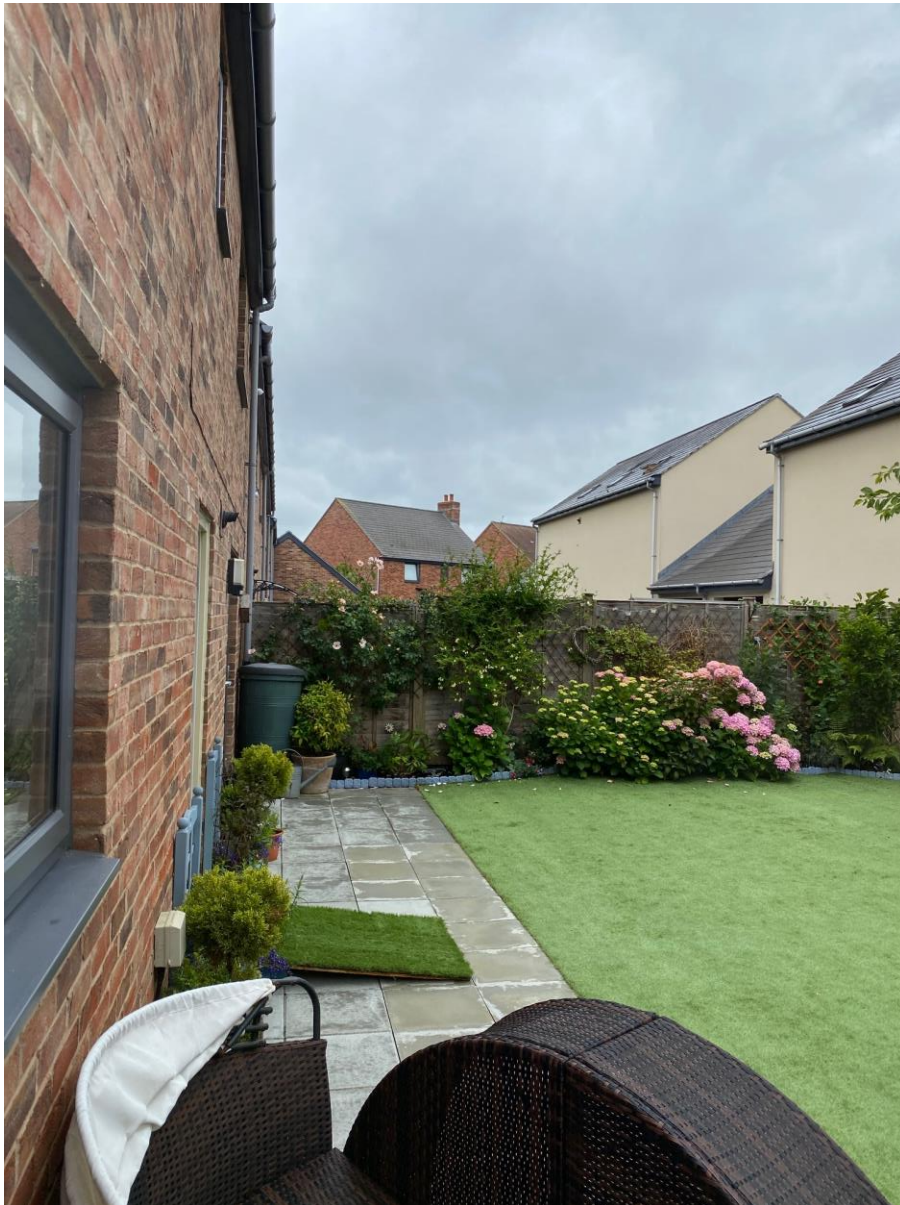
Photo 8: Side elevation. View from here would be the bifold doors:
