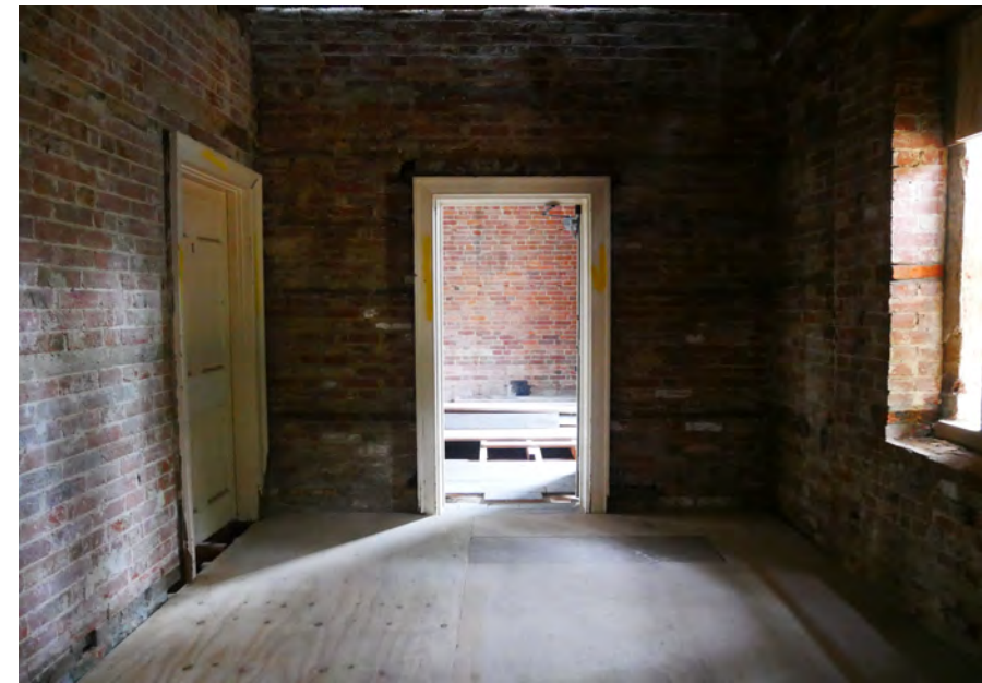
6. Exposed brickwork to south, east and west walls with view through to G4 - late Victorian Cross Wing.
