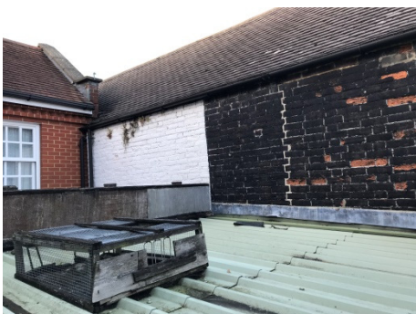
Junctions with the neighbouring property (party wall) where there is water ingress internally
