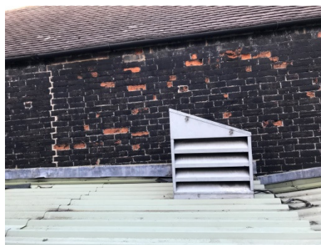
Junctions with the neighbouring property (party wall) where there is water ingress internally
