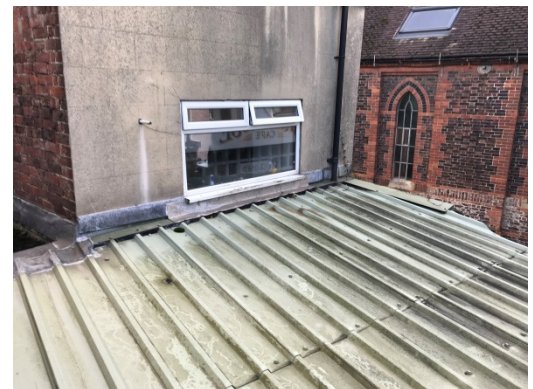
Existing junctions with the main building
