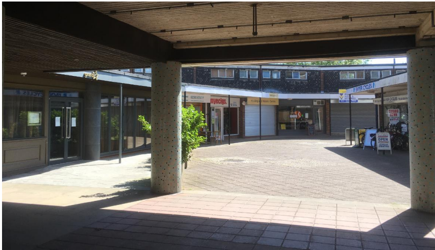
Figure 4 View East Through Undercroft from North Street
