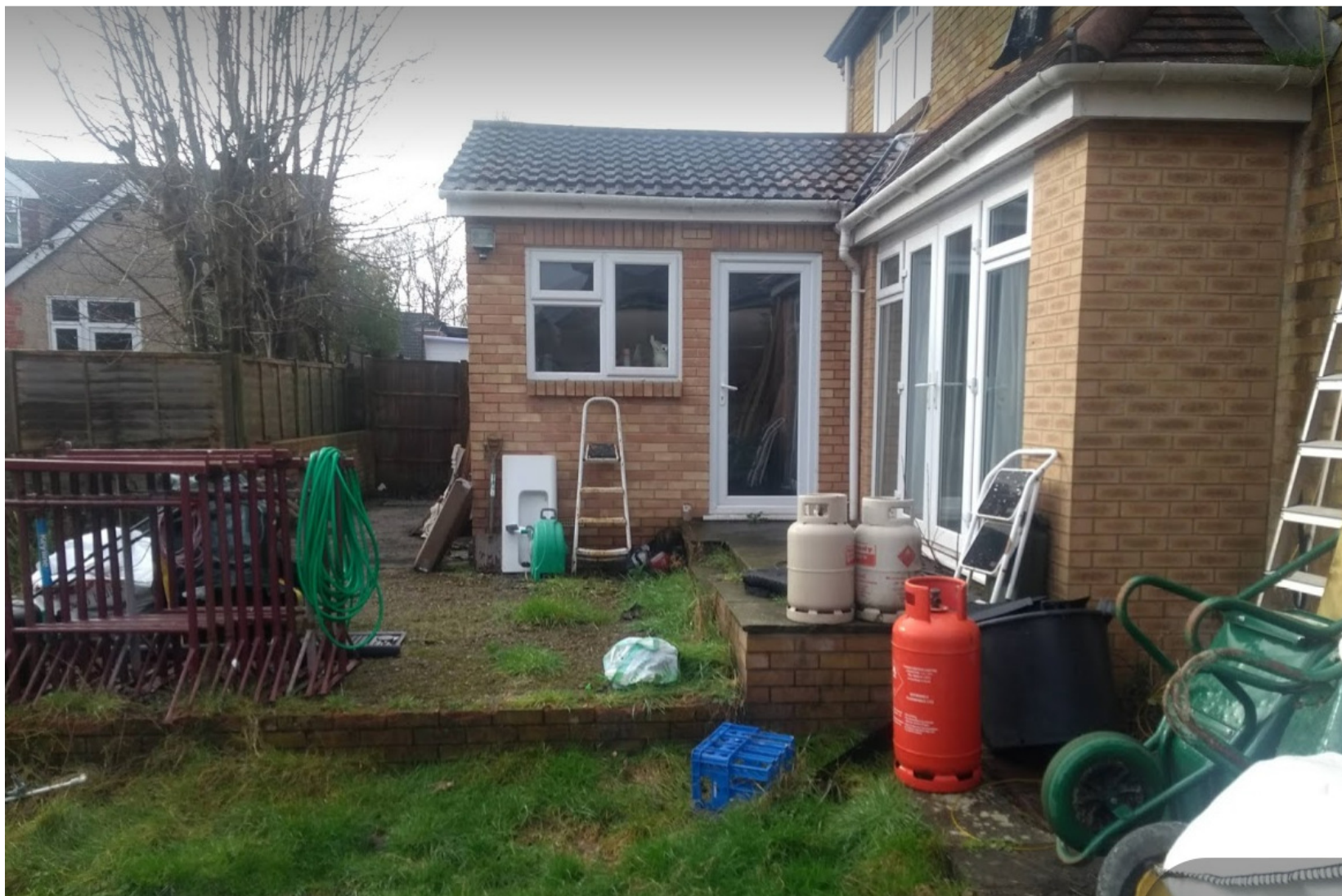
Rear patio of existing house
