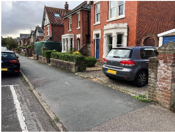
Figure 1, existing dropped kerb to 20 Grove Road.
