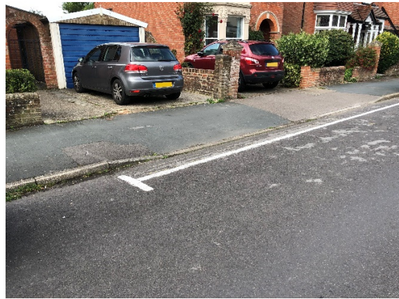
Figure 2, existing dropped kerb to 20 Grove Road.
