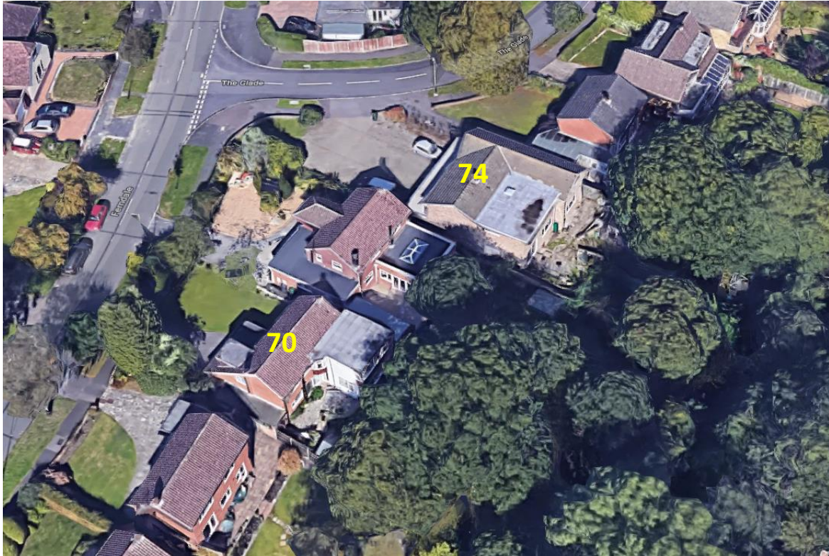
Figure 7 Aerial Photograph showing 2-Storey rear Extension Constructed at Nos 70 and 74 Ferndale
