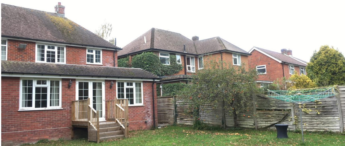
Figure 4 View of the Rear of No.62 and Adjacent Dwellinghouse No.64 Ferndale
