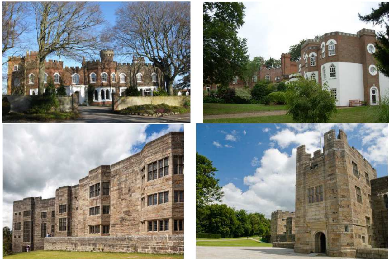
Figure 1.3 Existing Site Photographs
