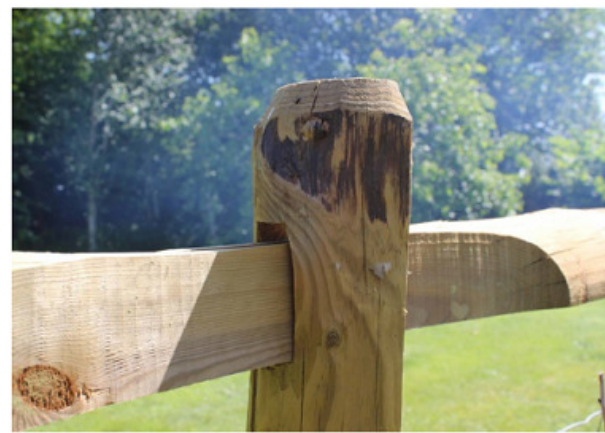
Morticed and tenoned rail and post joints
