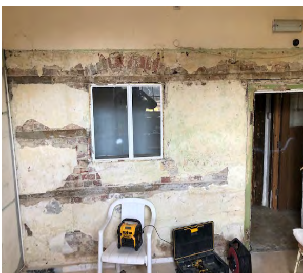
36. Inner south wall, single brick thick. Door and window to a former external passage.
