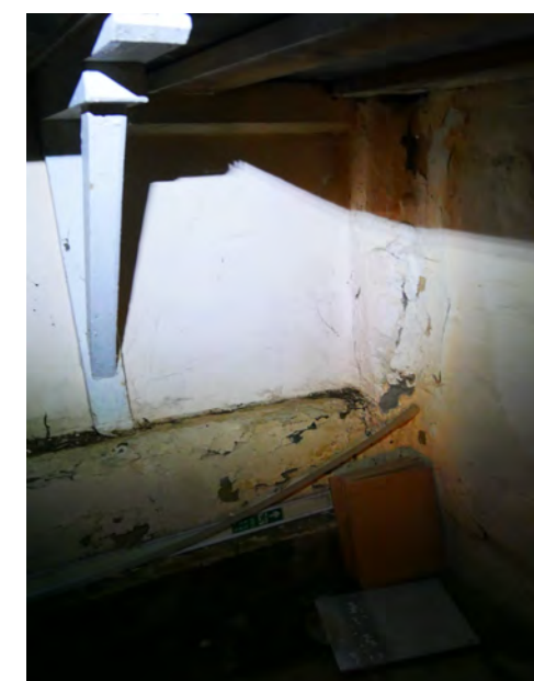
41. SE corner of G17 - the sole plate is clearly visible and is also evidence of the existence of the north bay.
