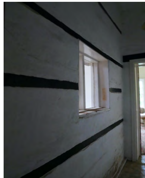
37. G15 - Former external wall to G16. Single brick thick and rudimentary dairy/agricultural form of construction.
