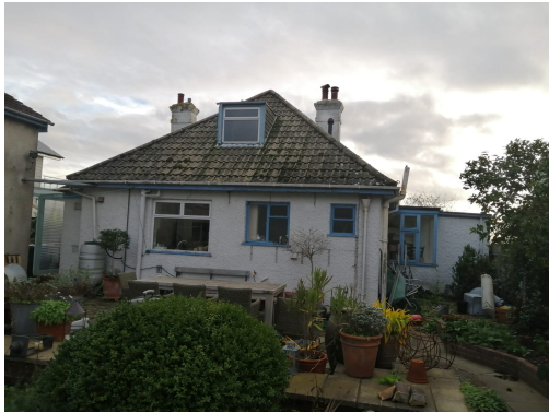
Figure 4. Northern elevation of Point View.
