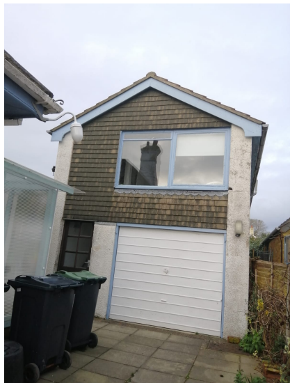
Figure 7. Southern elevation of the outbuilding at Point View.
