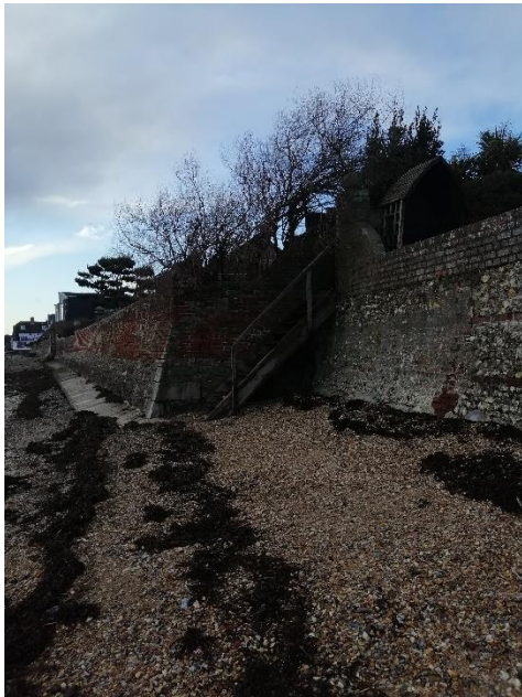
Boundary wall at 2 Swan Close
