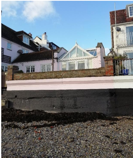
Boundary wall at 46 South Street
