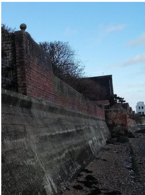
Boundary wall at 25 Tower Street
