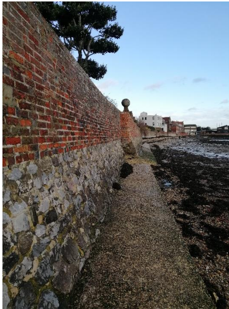
Boundary wall at 3 Swan Close
