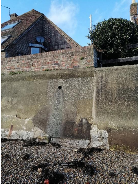
Boundary wall at 6 Seaview Terrace
