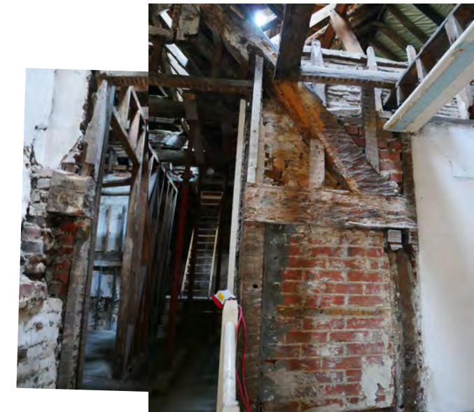
58. View to the south reveals the original wall plate, principal rafter and principal post. As the floors beyond have been raised, the door cuts through the end wall plate.
