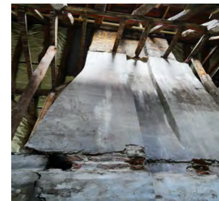
60. The original build had a stack but it has been increased in height correlating with roof changes.
