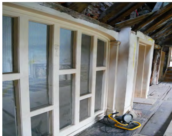
55. Brick above the wallplate relates to the roof over what became a parallel range.
