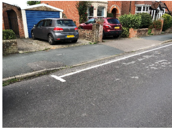
Figure 2, existing dropped kerb to 20 Grove Road.
