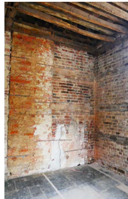
93a/b. South wall of FF15 with evidence of flue for FF13. Also potential evidence of a two stage build at first floor level. Note there is a partition line to the west of the door, not aligned with the paired beam above (reused).
