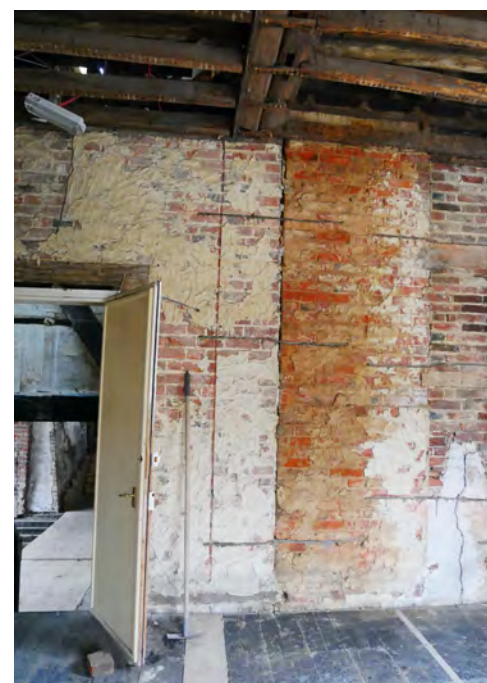
93a/b. South wall of FF15 with evidence of flue for FF13. Also potential evidence of a two stage build at first floor level. Note there is a partition line to the west of the door, not aligned with the paired beam above (reused).
