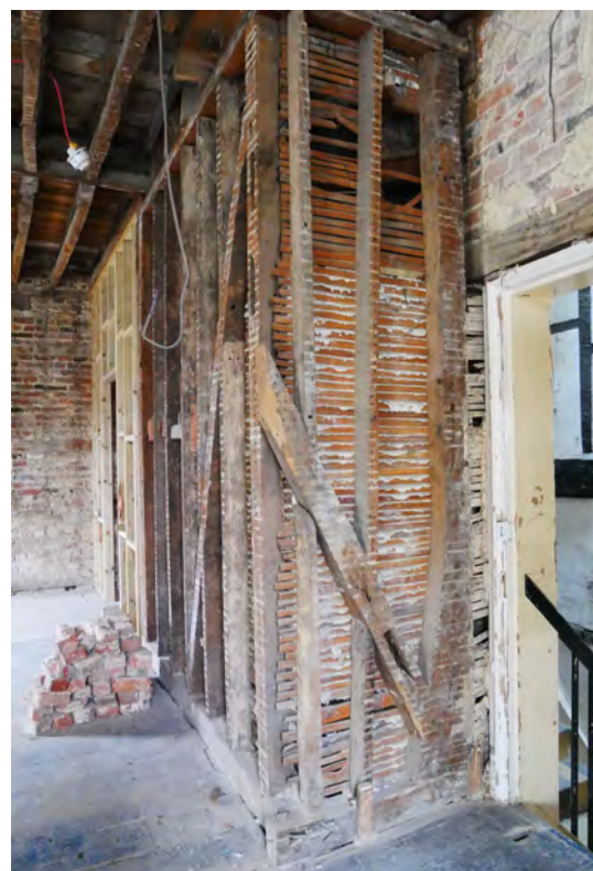
91. Stairs from FF14 to FF15 with later partition to accommodate landing. Note upturned 'swell' jowl to corner and reused rake. Softwood to east, more recent.
