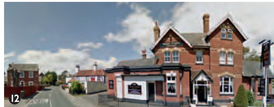
View of restaurant and public house on Station Road
