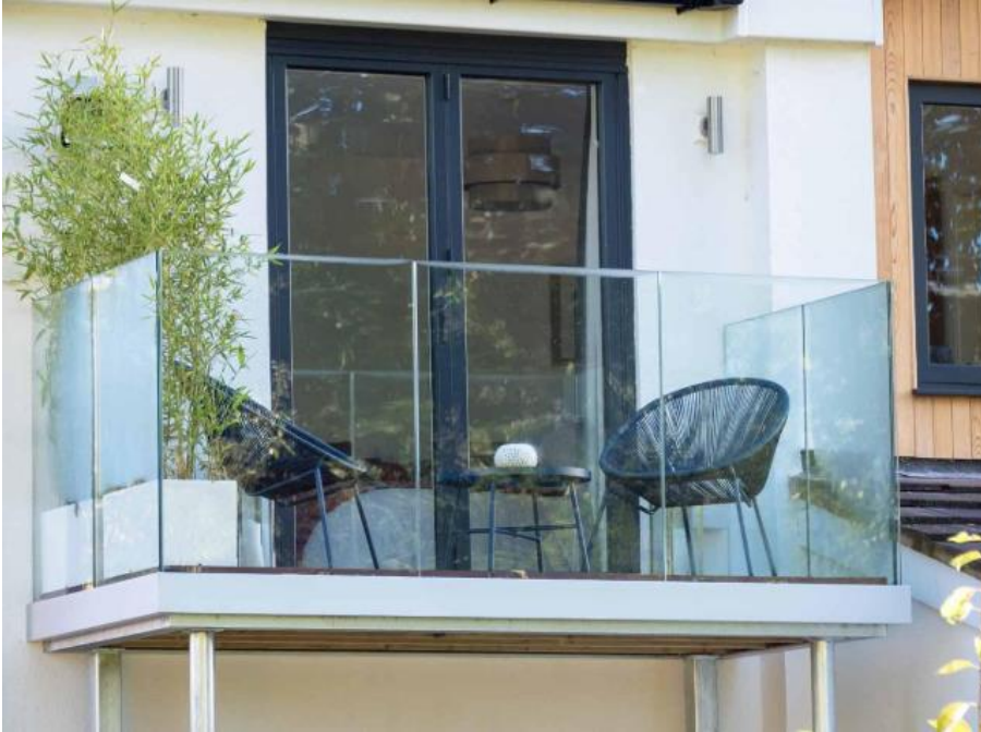
Example of contemporary, frameless, glazed balcony
