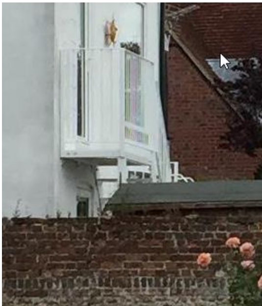
Existing balcony and external stairs to the courtyard garden
