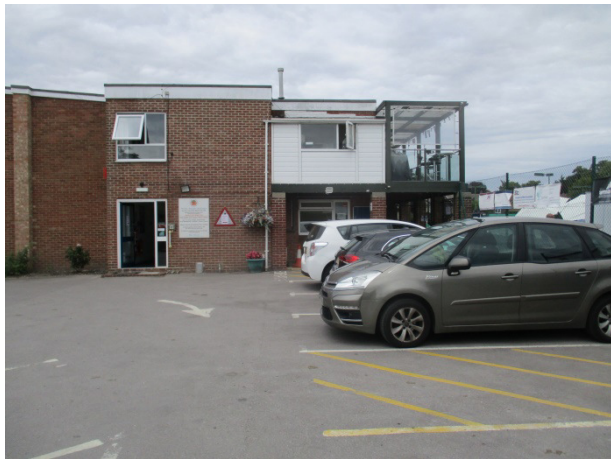
Fig 1: View of clubhouse entrance from car park
