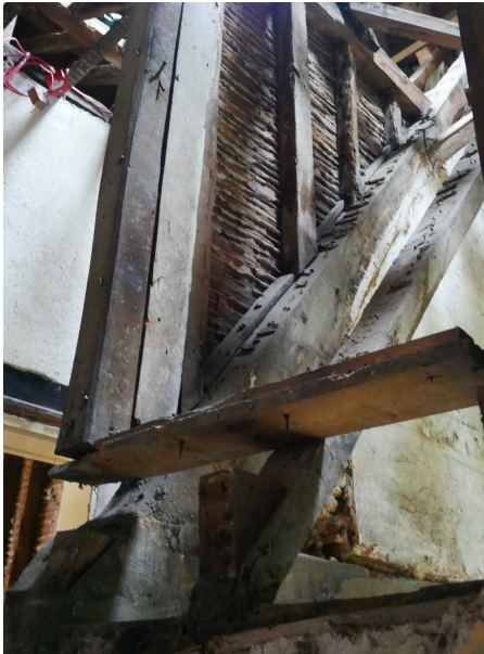
79a & b. East wall plate height with view of roof over middle bay. Shows evidence of fire damage, reuse added rafters along withraking shores. Rafters are also added to increase the height over the main range. Ashlars indicate ceiling height to FF12/13 raised. The principle post and rafter can be seen as the divide for the original north bay. Studs added to create FF14 partition. Roof over main chamber - rafters are bridle jointed at apex. Marked II and II.
