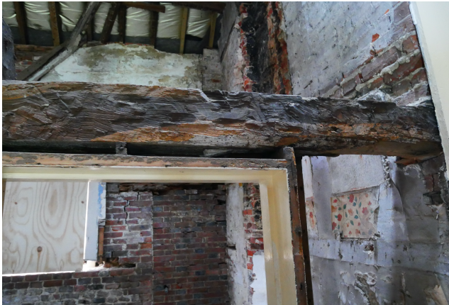
81. West wallplate 'interior' face, at pt where the 3rd nrth bay existed. Note evidence of bay window. Former fireplace & flue removed in past.
