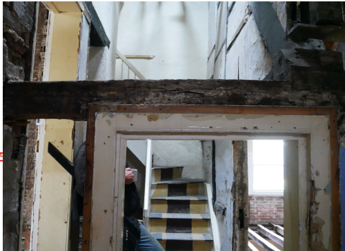
80. West wallplate to 'ghost' north bay and FF14. Note that box frame is visible to the stairway.
