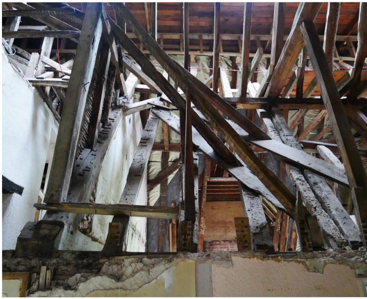
79a & b. East wall plate height with view of roof over middle bay. Shows evidence of fire damage, reuse added rafters along withraking shores. Rafters are also added to increase the height over the main range. Ashlars indicate ceiling height to FF12/13 raised. The principle post and rafter can be seen as the divide for the original north bay. Studs added to create FF14 partition. Roof over main chamber - rafters are bridle jointed at apex. Marked II and II.
