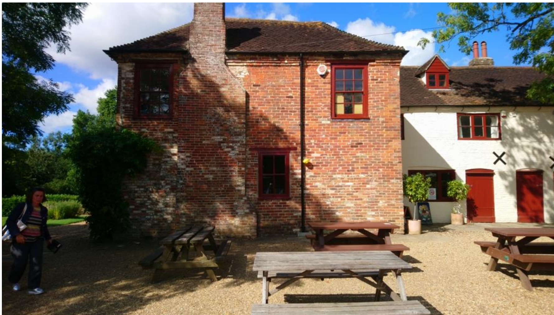
East Elevation View of Courtyard
