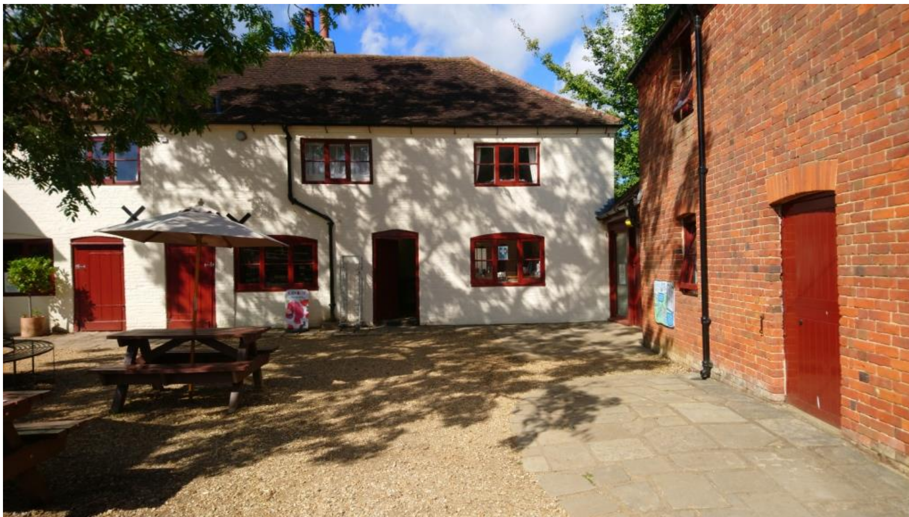
East Elevation View of Courtyard
