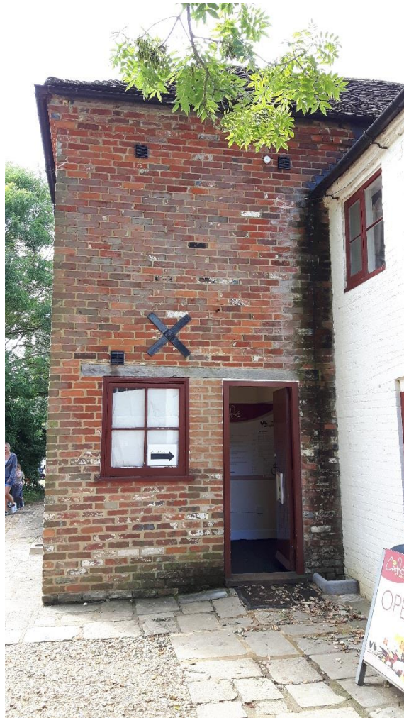
View of Entrance door
