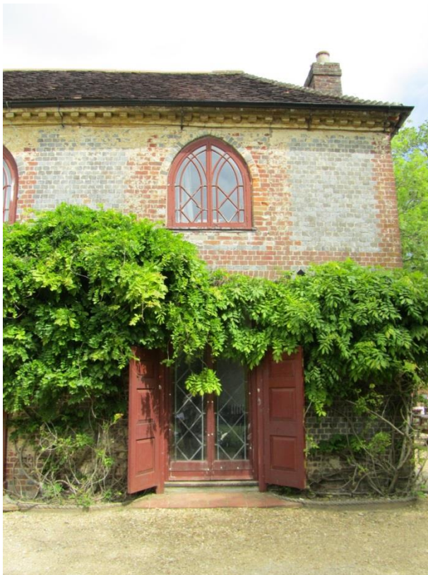
Fig 4. Current View of South elevation of the Farmhouse
