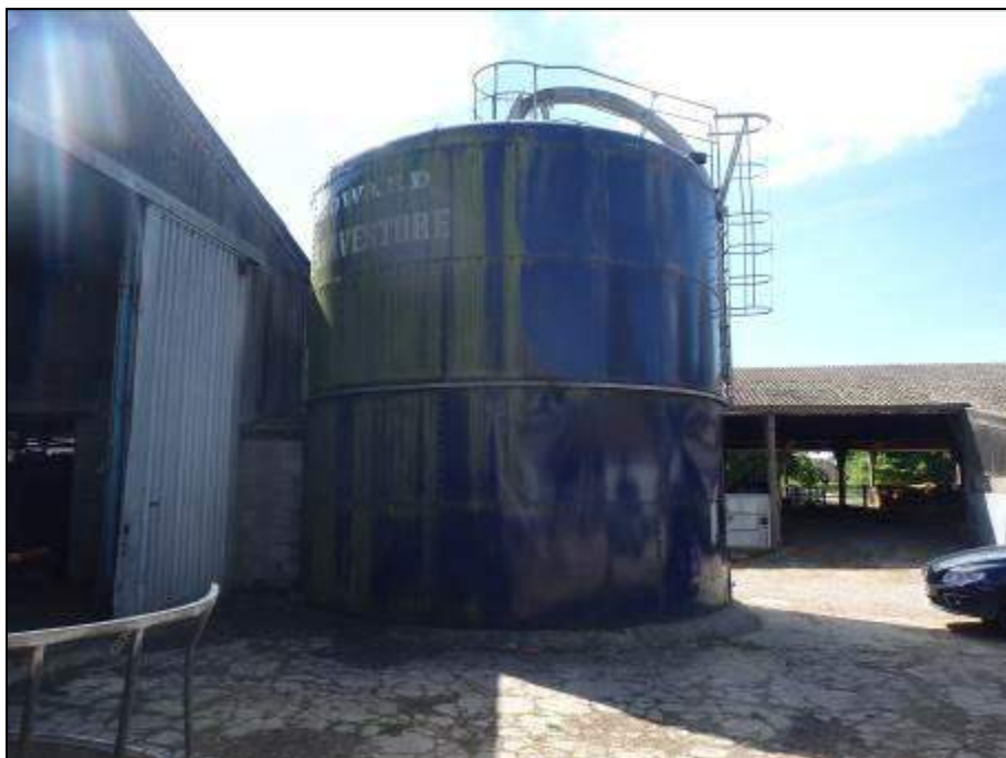
Photograph 9 Showing the adjacent silo and hay barn
