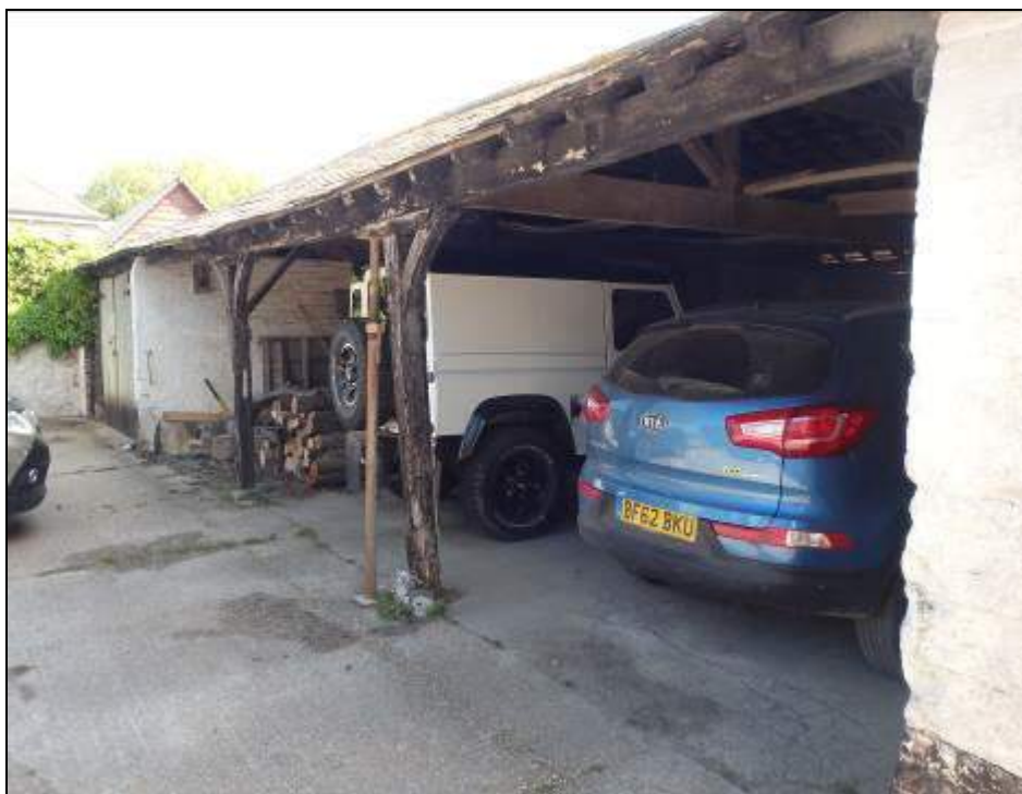
Photograph 2 Showing the former cart-shed on the western section of the site
