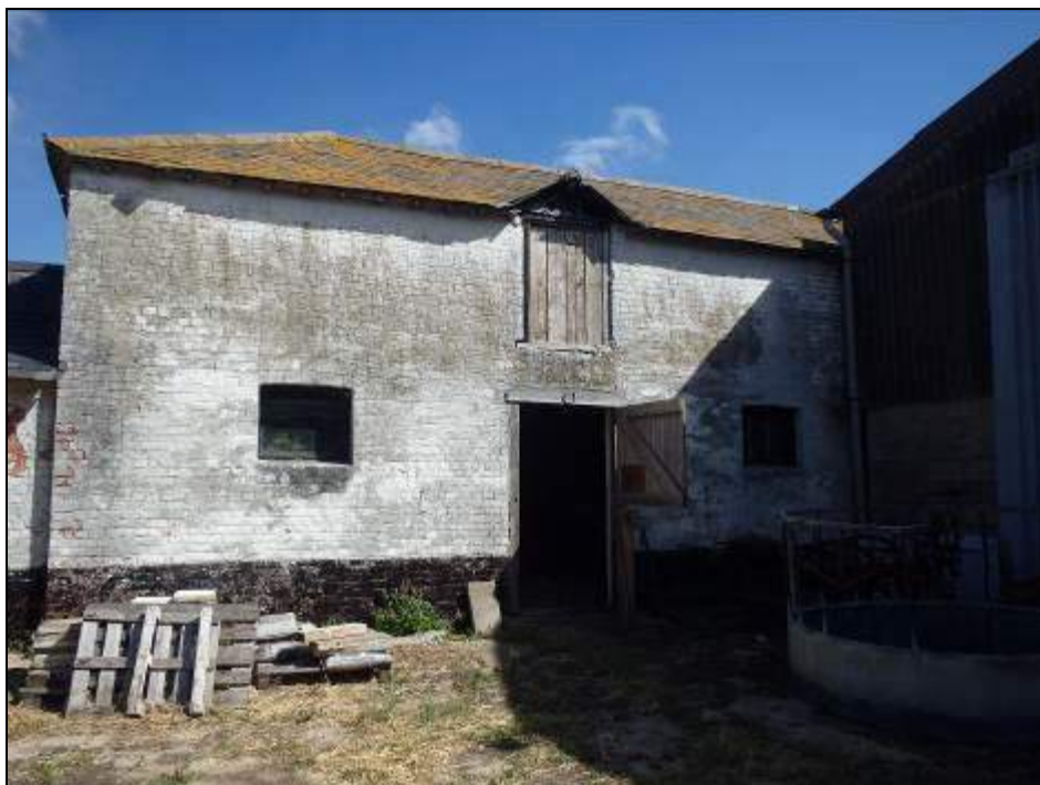
Photograph 7 Showing the eastern-most section of the subject building
