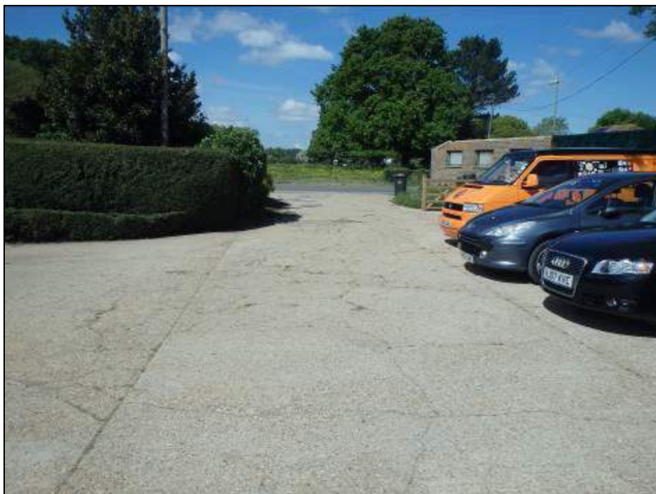
Photograph 1 Showing the entrance onto the site
