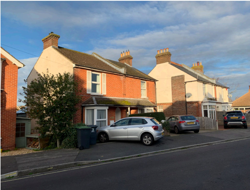
5 & 7 St James Road - East elevation
