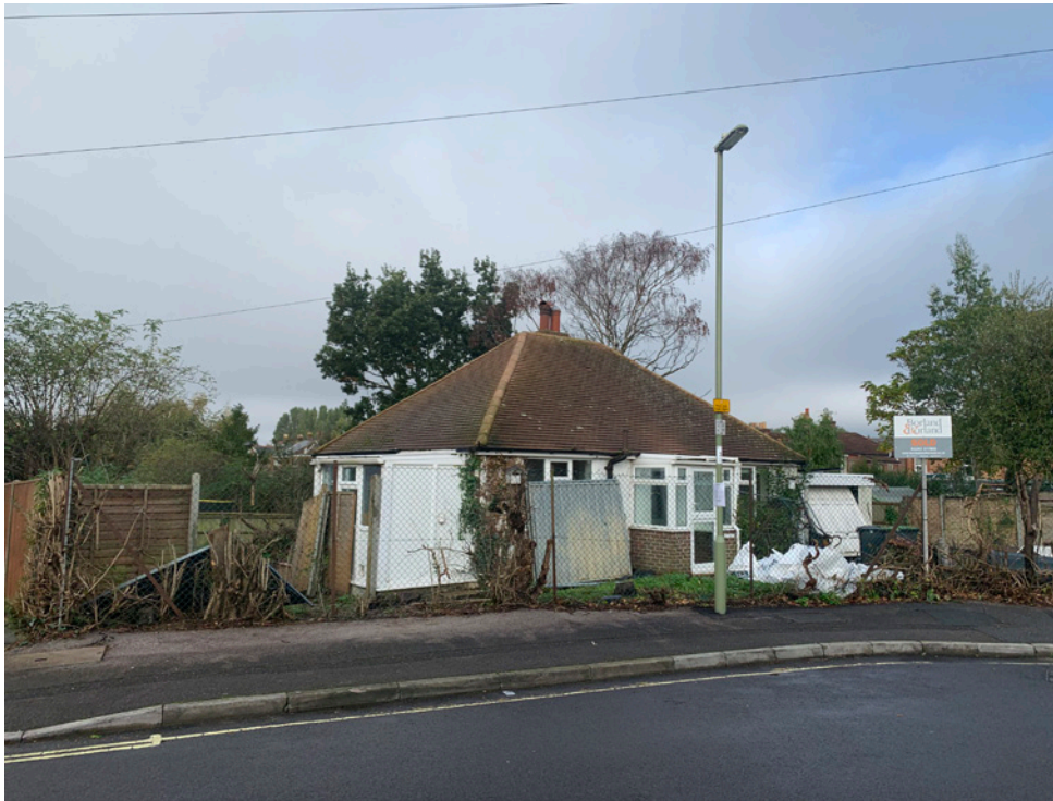
1A St James Road - View from East
