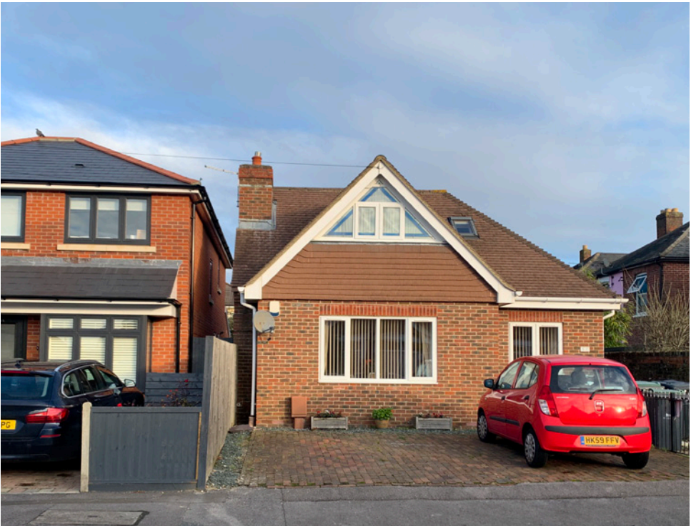
1F St James Road - South elevation (flat fronted gable)
