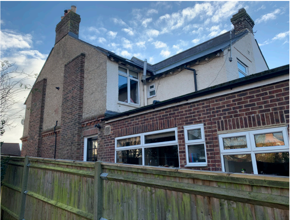
1 St James Road - Neighbouring two storey property with a single storey rear extension
