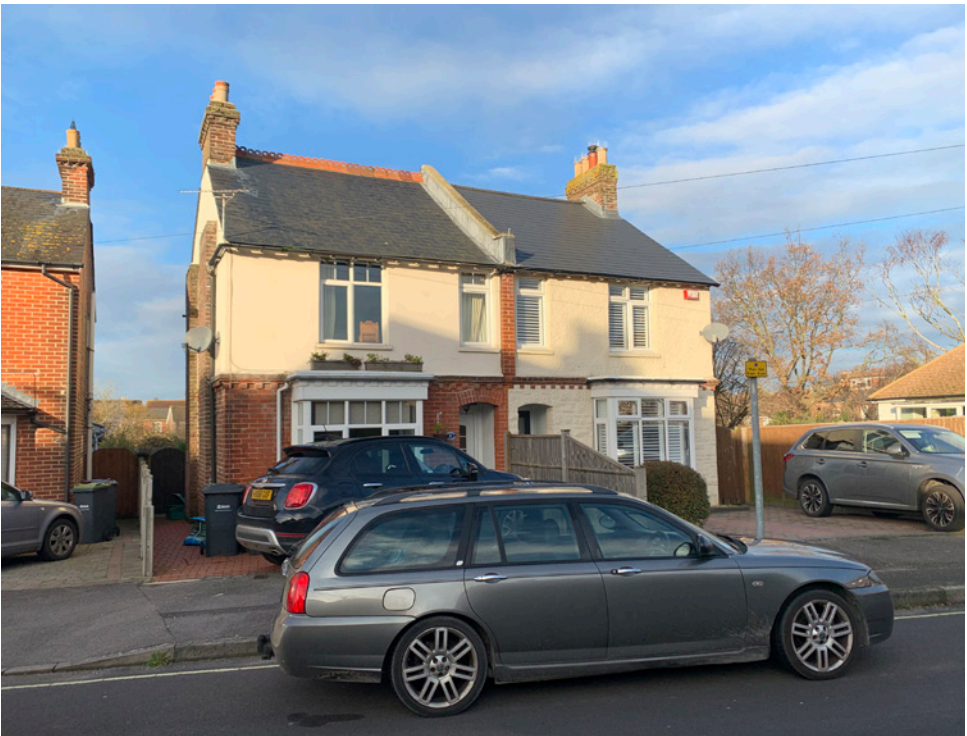
1 & 3 St James Road - East elevation
