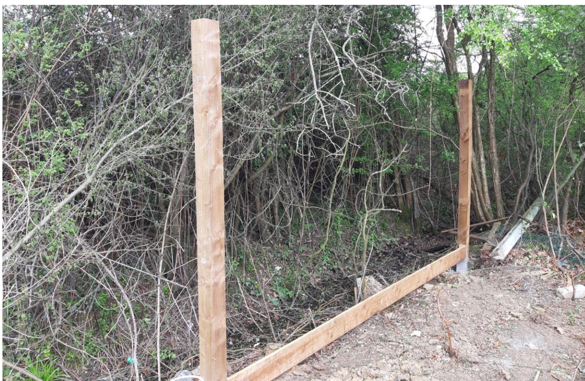
Photo 2: Boundary fence being erected
