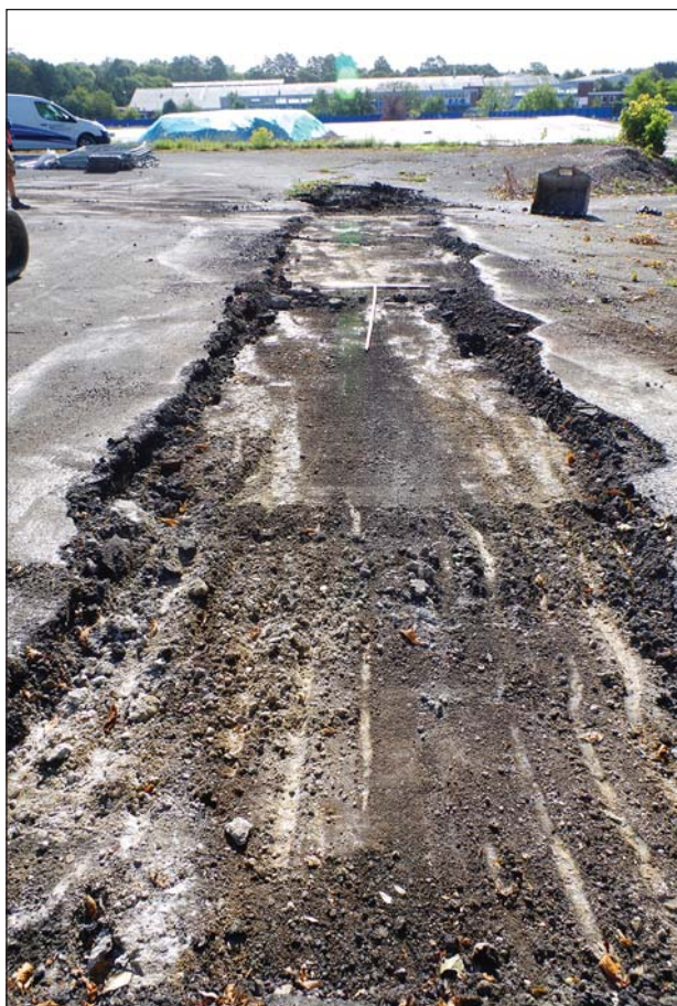
Plate 1: Trench 5 viewed from the north-west showing concrete 502 (1 x 2 m, 1 x 1 m)
