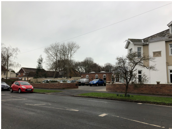
The site, viewed from the northeast, on Beech Road.
