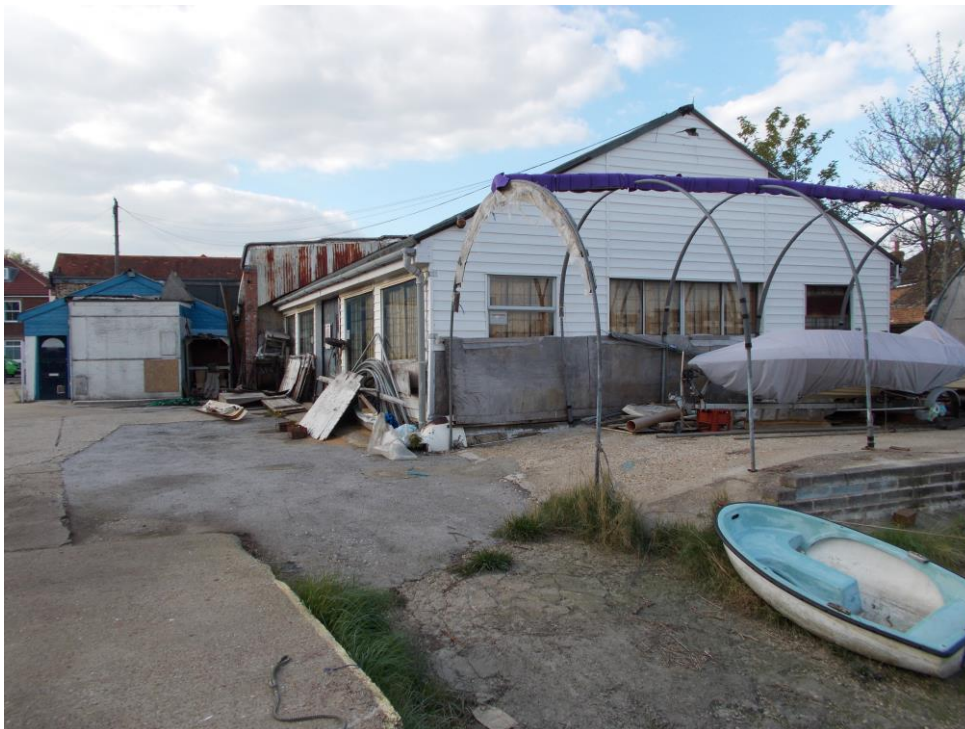
Figure iv. View from the slipway showing unkempt appearance.
