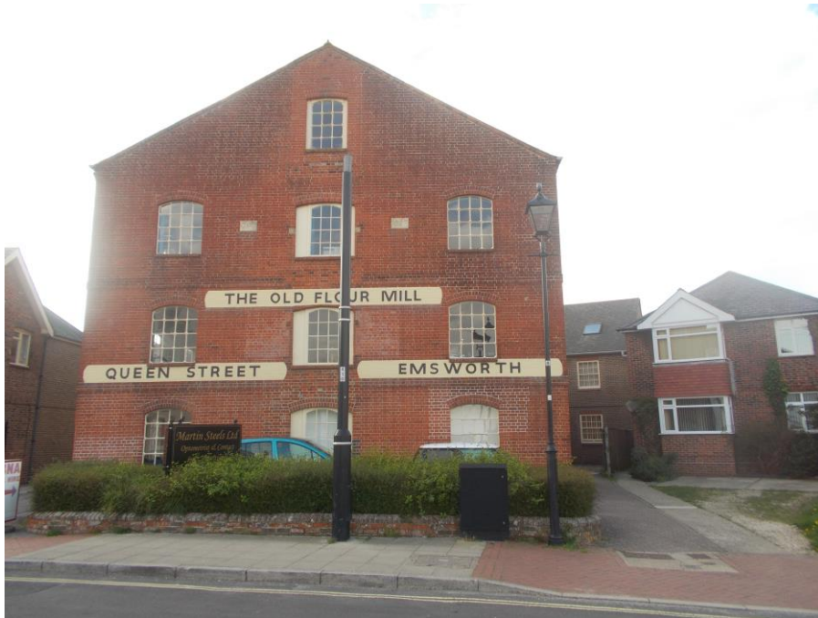
Figure vii. The Old Flour Mill sits opposite and slightly west of the site.
