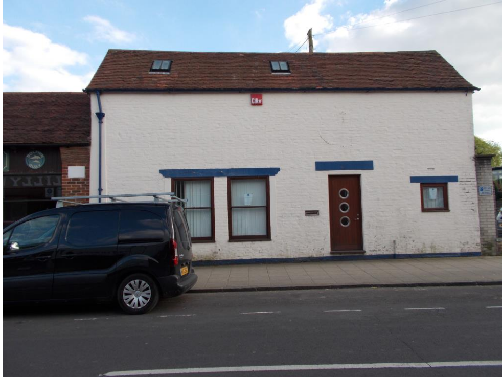
Figure i. 31A Queen Street, showing the much altered frontage.
