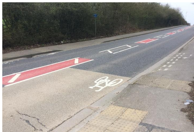
Photograph 11: Cycle Infrastructure along Crookhorn Lane
