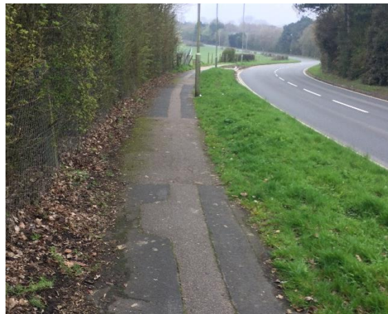
Photograph 1: Pedestrian Infrastructure along College Road
