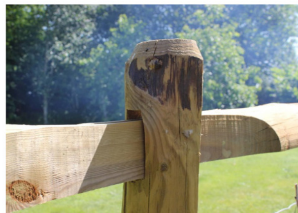
Morticed and tenoned rail and post joints
