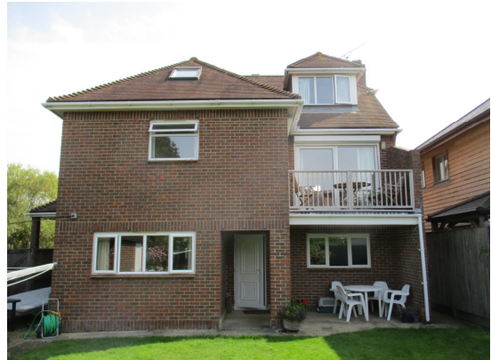
Fig 2 – View of the rear of the property
