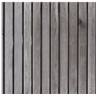
Fig 5 – Example of vertical Siberian Larch cladding.
