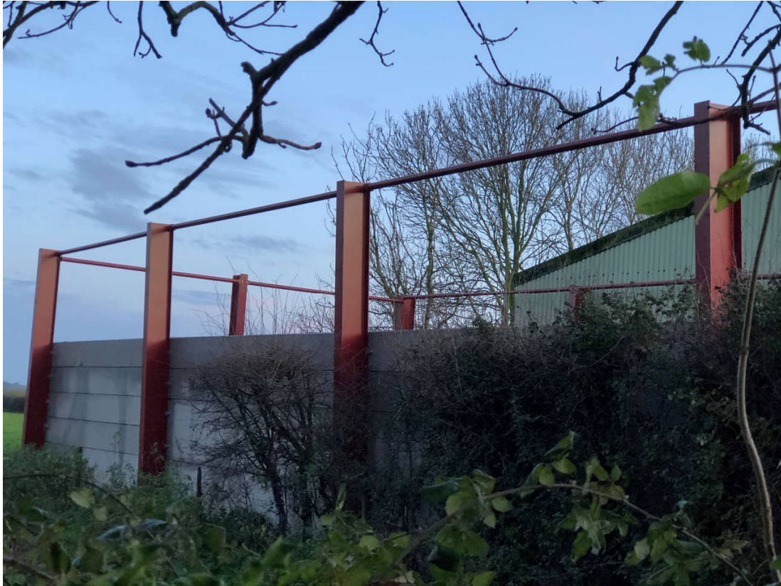
VIEW AT GARDEN CORNER
