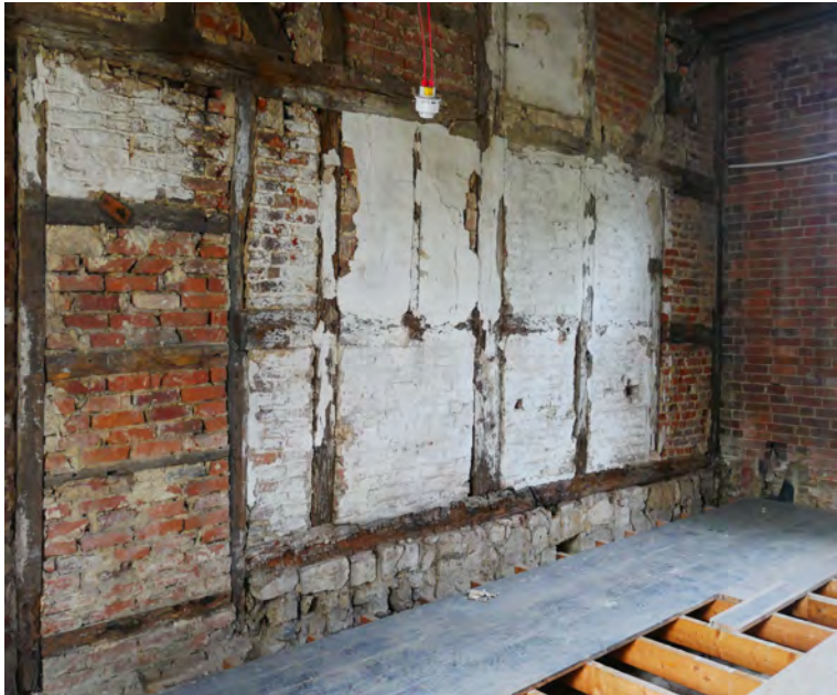
11. Timber-box frame to C16th 'end' bay with evidence of former door and window. Masonry plinth below cill plate. Evidence of cement mortar used for repairs and repointing.
