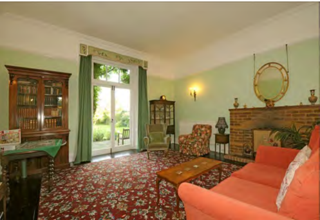
French doors and fanlight to G4 (replacement approved). Brick fireplace, skirting boards, picture rail and coving visible (Source: Zoopla).
