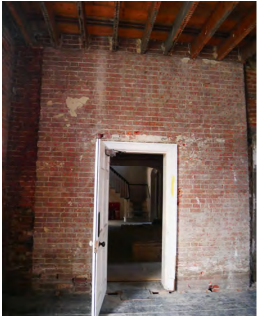
10. Exposed brickwork to NW corner. This shows the point where the Late Victorian south cross-wing range was added.
