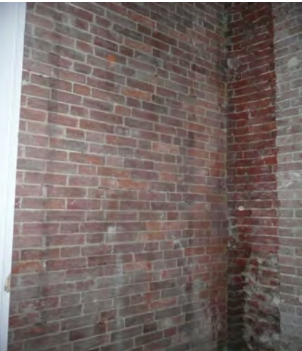
9. Exposed brickwork to NW corner. This shows the point where the Late Victorian south cross-wing range was added.
