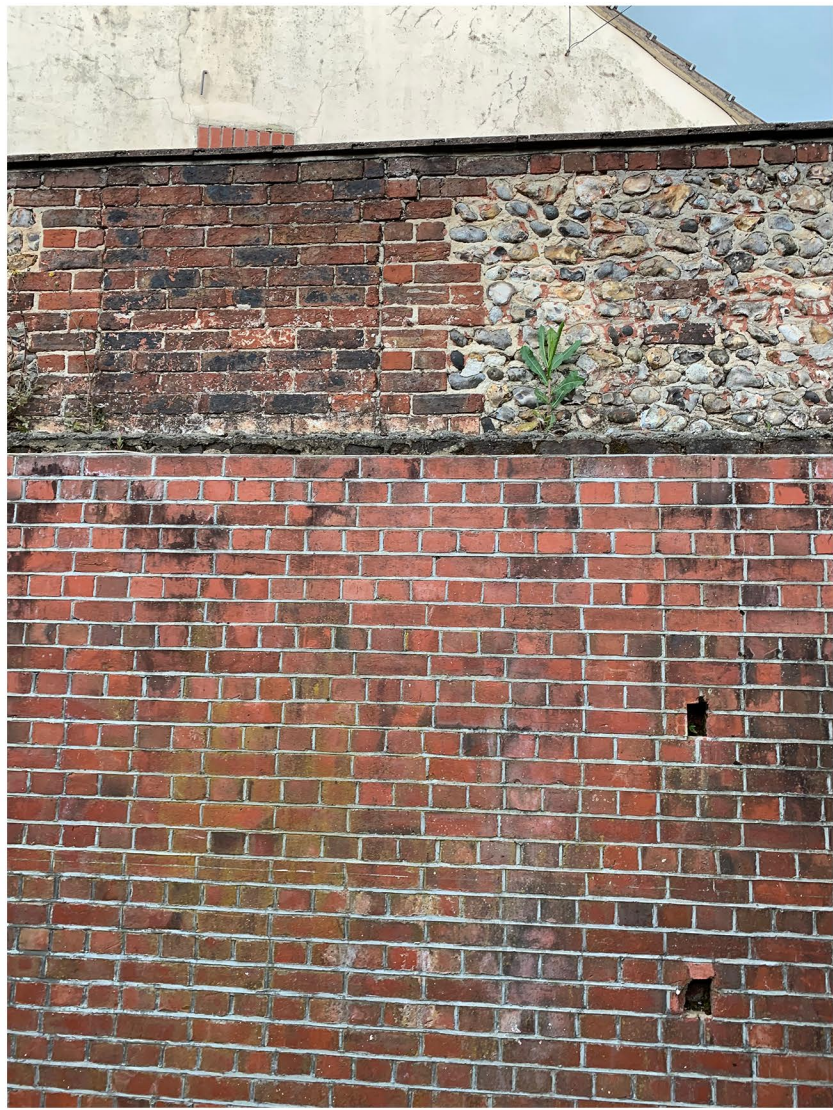
EXISTING BRICKWORK WALL TO BE CLAD
