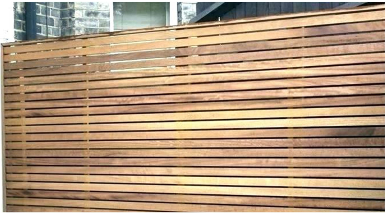
SLATTED TIMBER CLADDING TO REAR WALL
