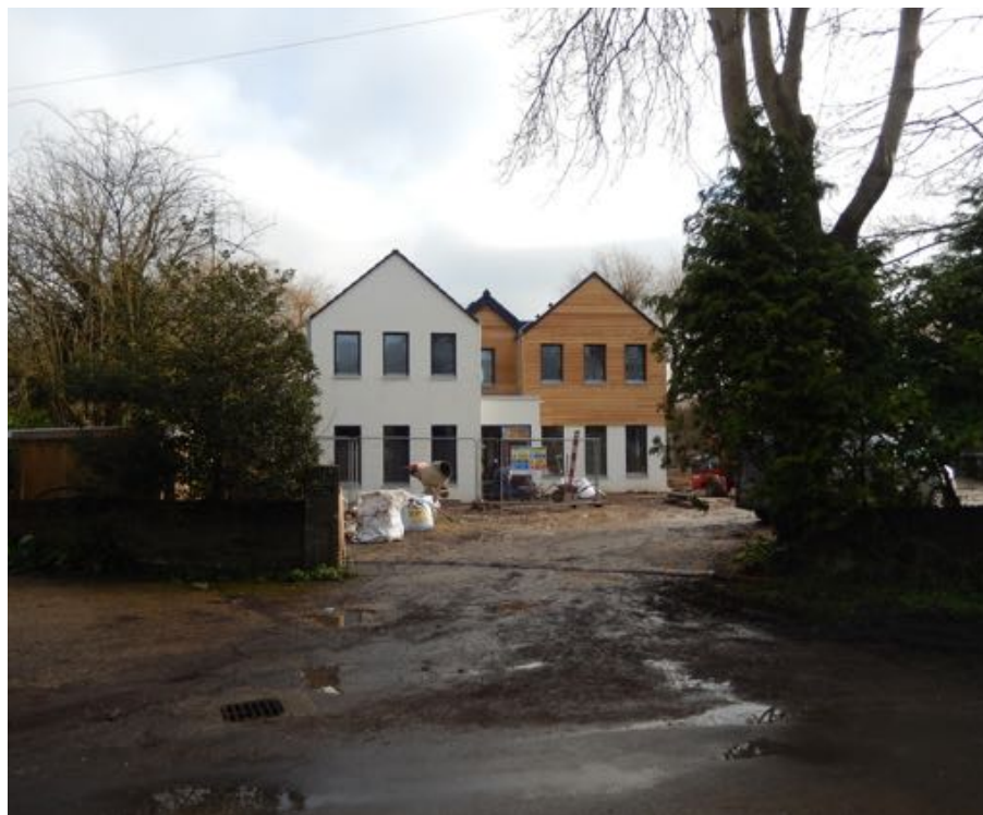
A new house under construction at 11 Lower Road ix
