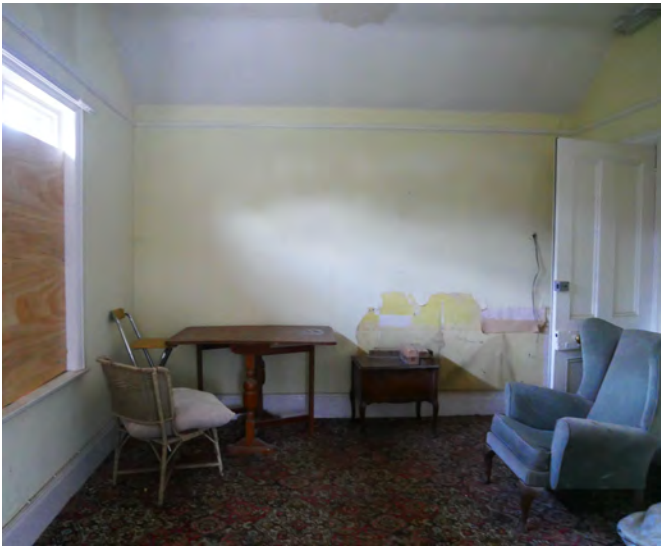
42. South inner facing wall of G18. LBC has been granted for new French Doors to lead onto the terrace.
