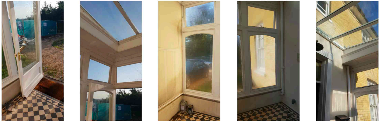
Photographs showing room 1 (porch)
