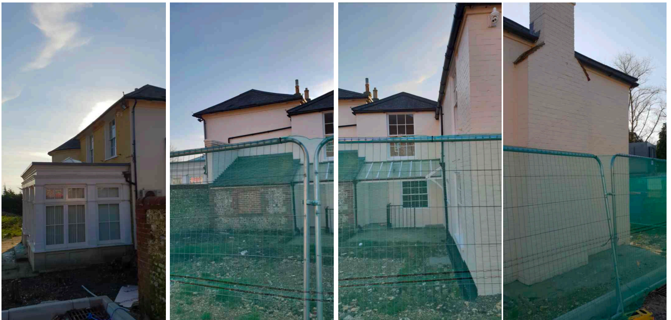
Photographs showing north elevation
