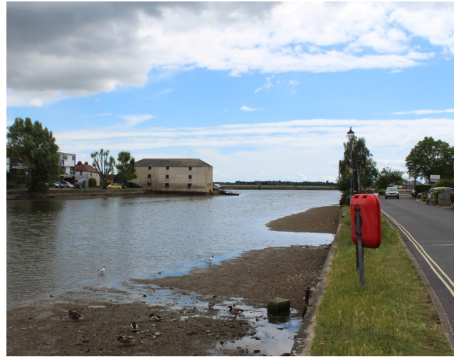
Photograph B. Slipper Mill Pond within Emsworth Conservation Area.
