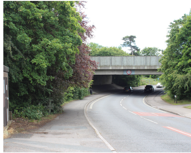
Photograph K. A27 passing over main road namely North Street to the south of the Site.
