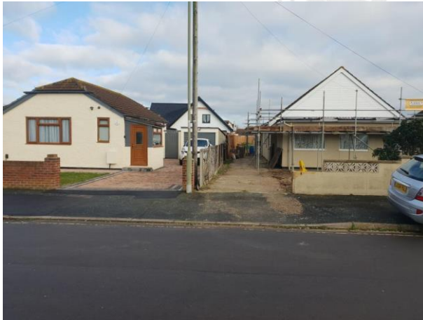
View of 16 Eastoke Av. from 5 & 7 West Haye Road
