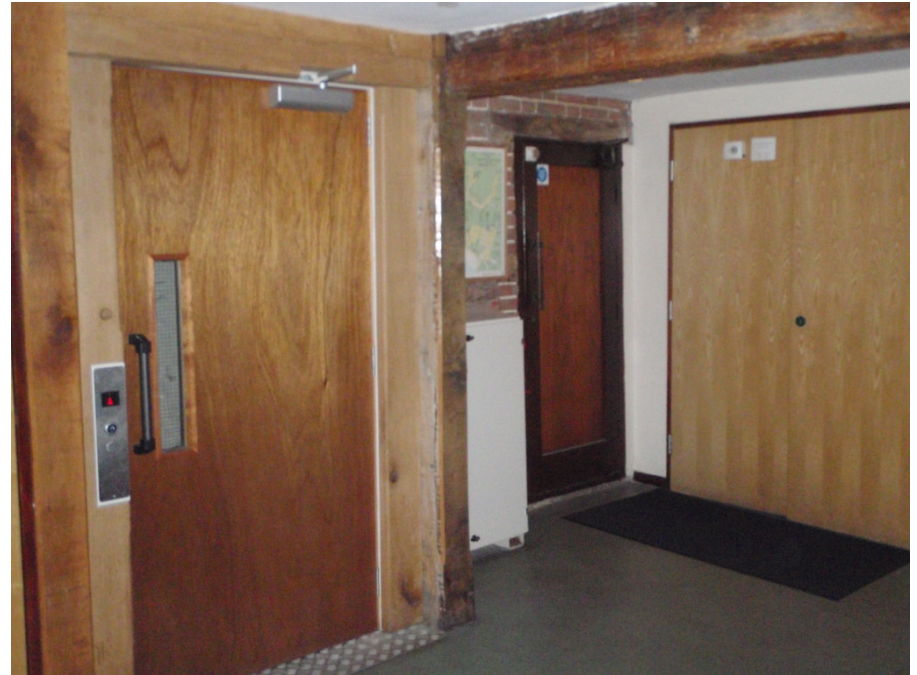
2. Lobby outside toilets.
