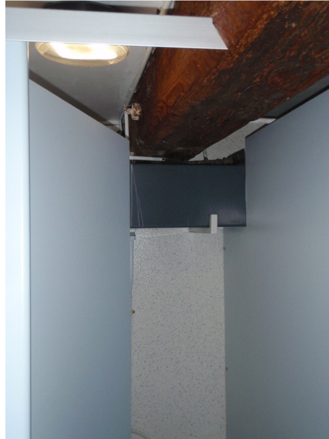
14. Exposed beam within the female toilets.
