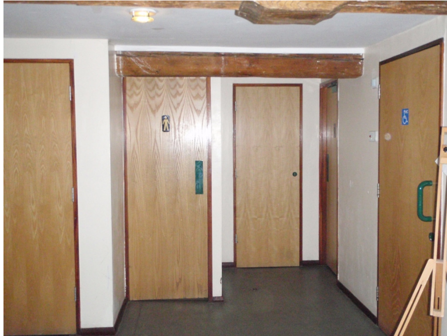
3. Lobby outside toilets.
