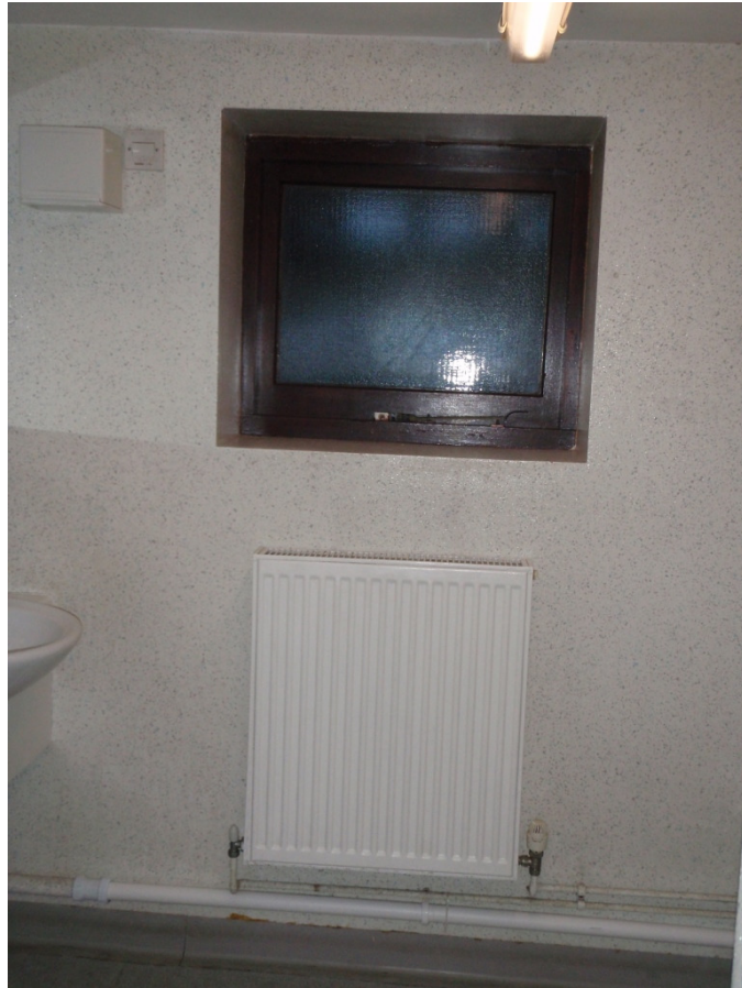
9. Part of the male toilets that will form part of the proposed galley area.
