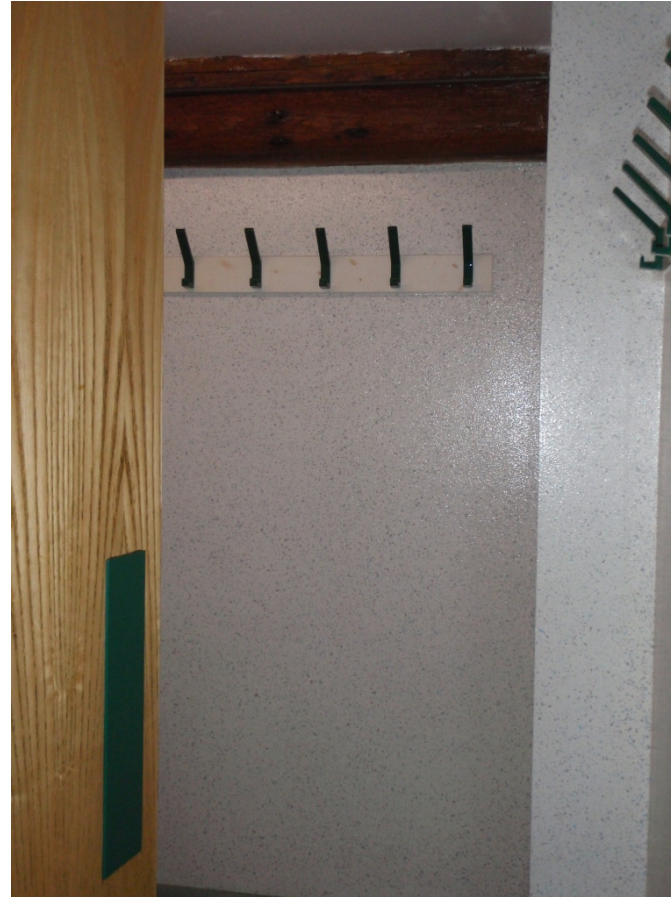
6. Dividing wall within male toilets, exposed beam above partition wall.
