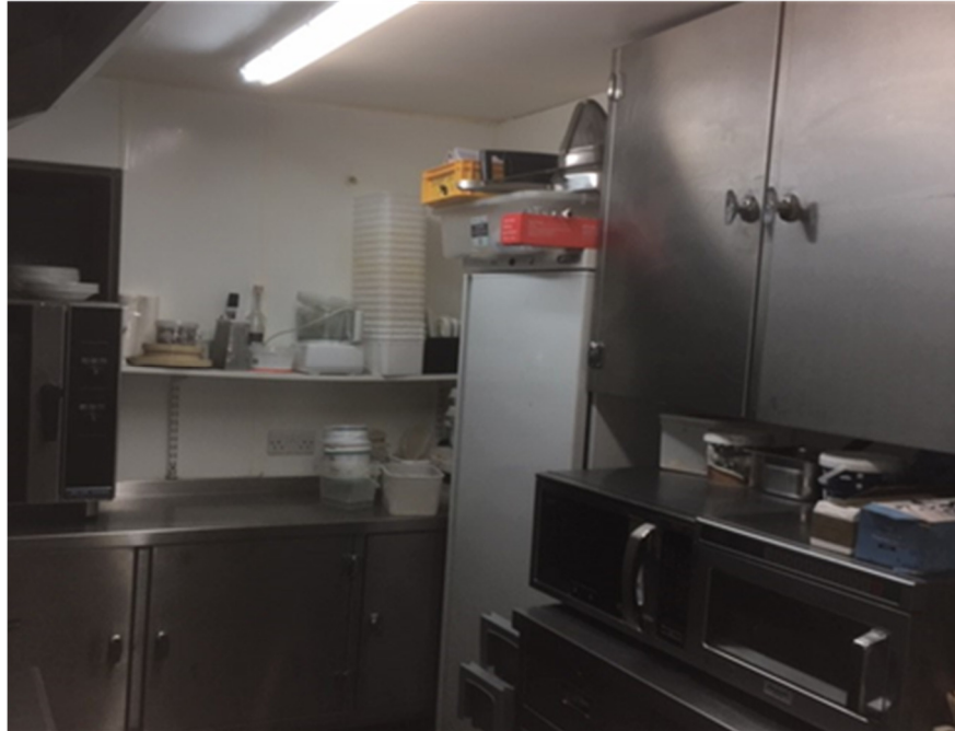
15. Recessed section of wall to be removed and new opening formed behind fridge.
