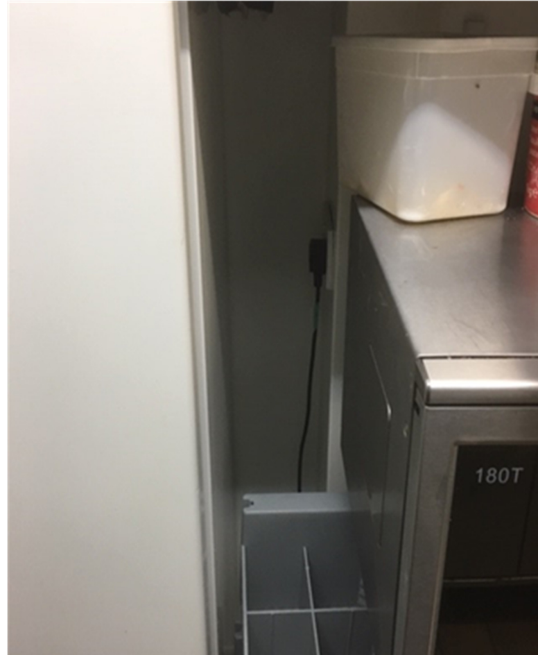
16. Recessed section of wall to be removed and new opening formed behind fridge.
