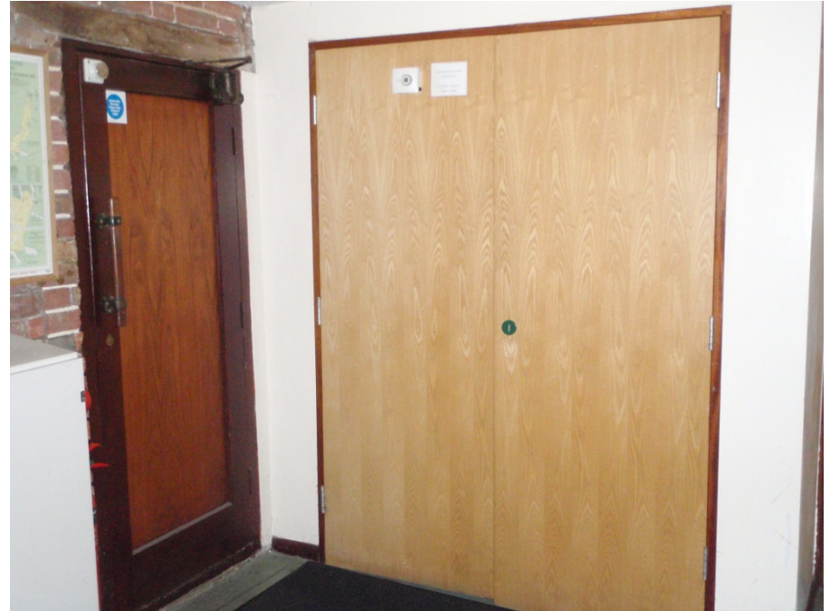
4. Lobby outside toilets.
