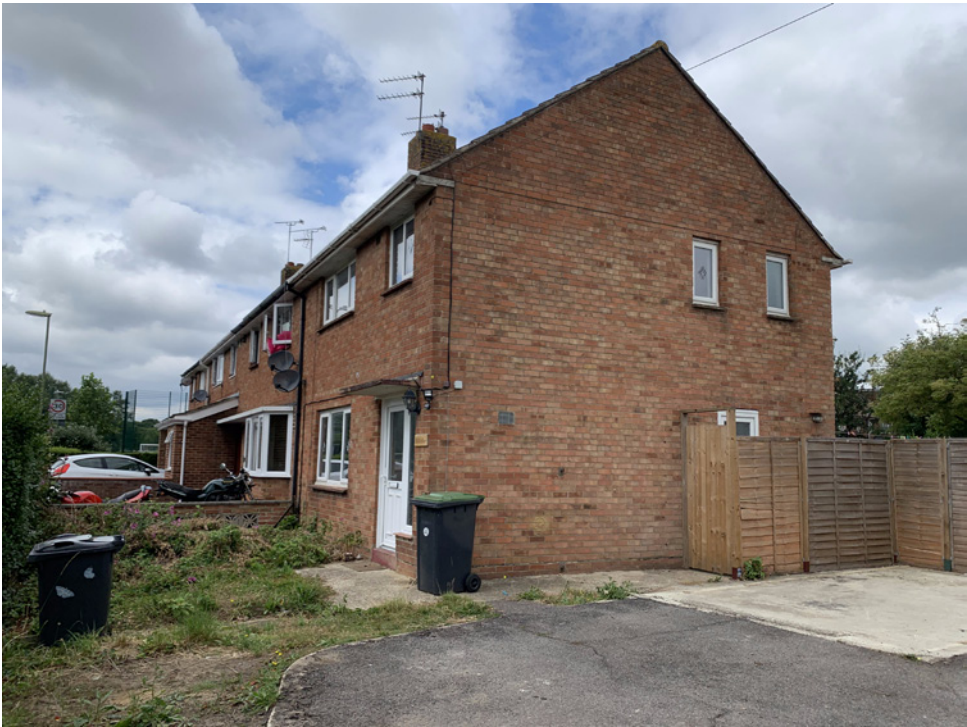
16 Selborne Avenue - View along western boundary.
