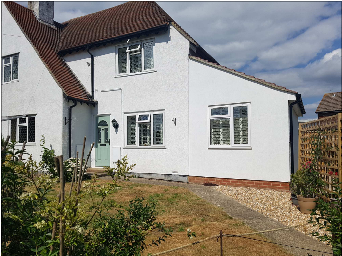
Alternative view into garden from road, showing lack of privacy as a result of the gap in the hedge
