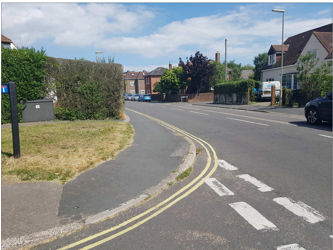
Car view down road. This will be improved by the removal of the hedge.
