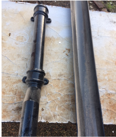
Section of guttering and downpipe still in situ. Guttering and downpipe removed, repaired and ready for reinstatement.
