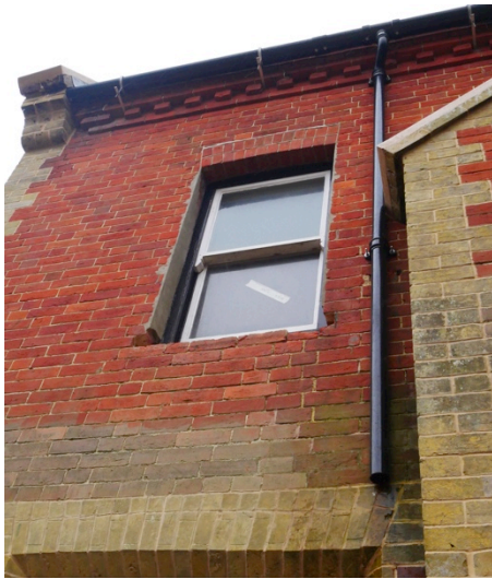
Section of guttering and downpipe still in situ. Guttering and downpipe removed, repaired and ready for reinstatement.
