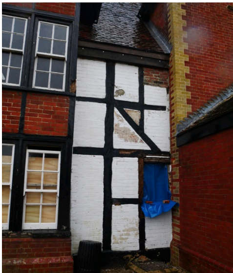
Eaves board to which guttering was attached to rear elevation. Also runs of guttering attached to eaves board of full height square.
