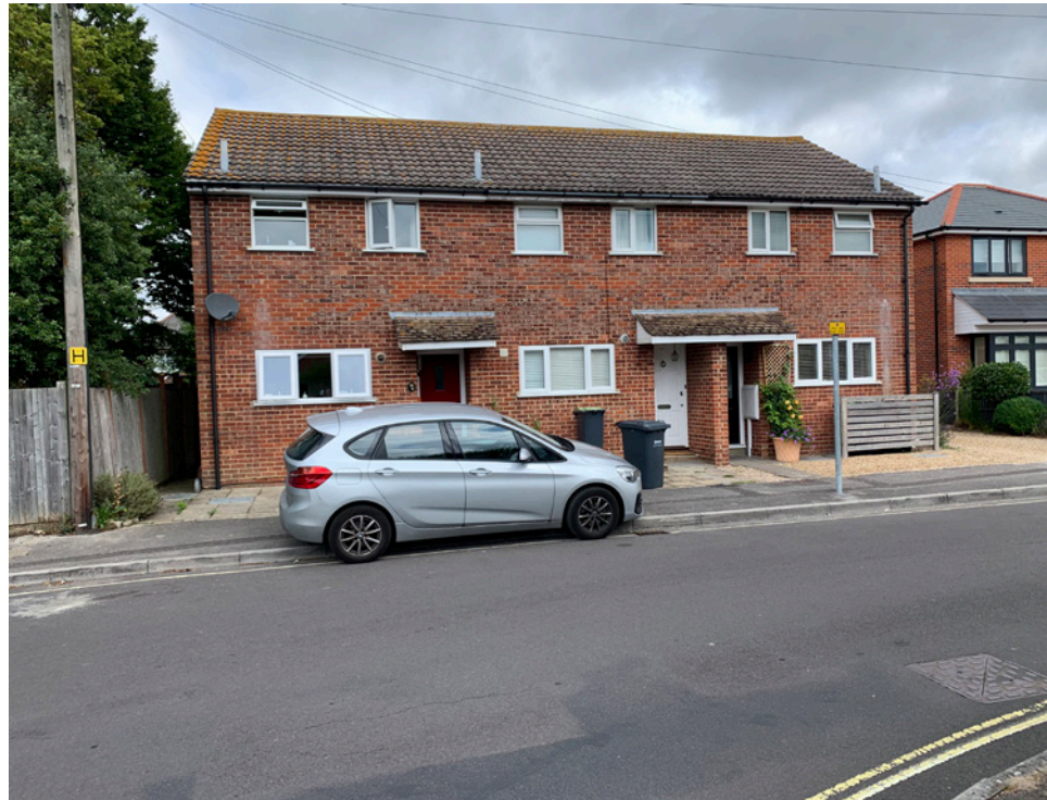
St James Road - Showing mixture of fencing & hard landscape
