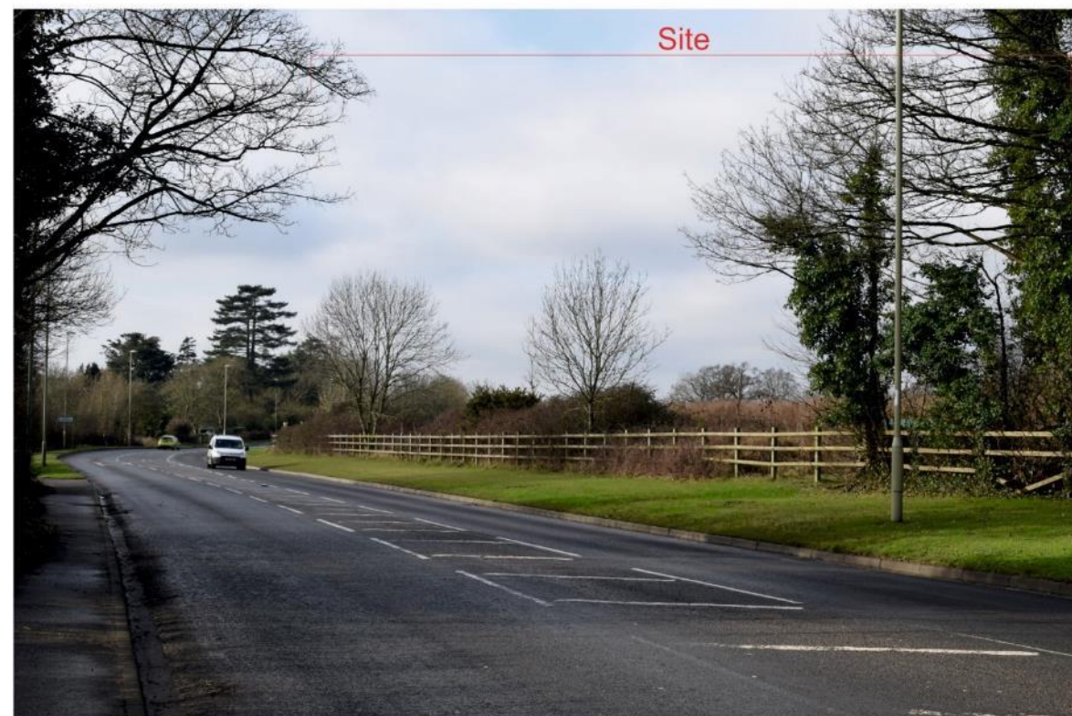
Viewpoint 9: S/E Photo taken from the south of Barton's Road opposite the Spire hospital entrance road looking west down Barton's Road and northwest towards the site. The site's ground plane is not visible due to the intervening trees and vegetation even in winter, though the tops of the mature oaks within the site are visible and proposed housing would also be visible.
