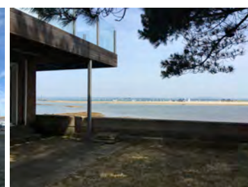
04 Harbour Wall as seen from inside of property No.36a
