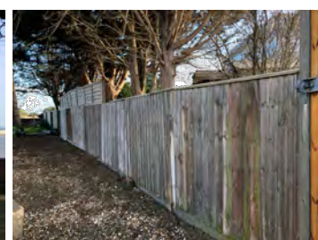
05 Existing fence and screening towards No.36
