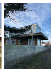
03 Harbour Wall from seaside
