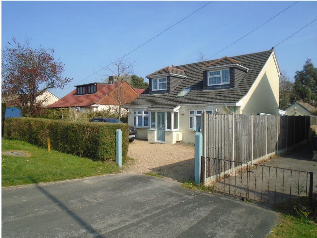
Figure 3. Nos. 90 and 92 London Road with rooms in roofspace.
