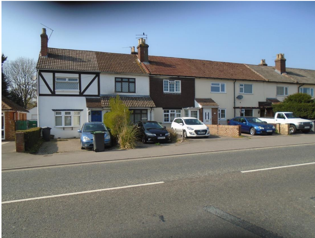
Figure 2. Two-storey terraced dwellings opposite the application site.
